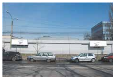
BANNER DISPLAY ON ROMEXPO HEADQUARTER FACADE
